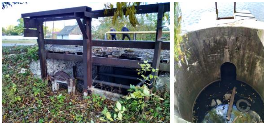
Fig. 7. Damaged spillway structure and empty spillway shaft at ponds in the riverbed of the Pavolochka river
